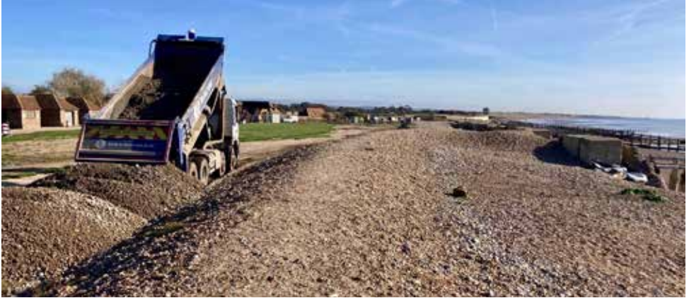
(Above and below) Shingle material being positioned on the flood defence by Environment Agency officers.
