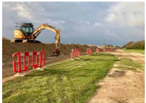
(Above and below) Shingle material being positioned on the flood defence by Environment Agency officers.
