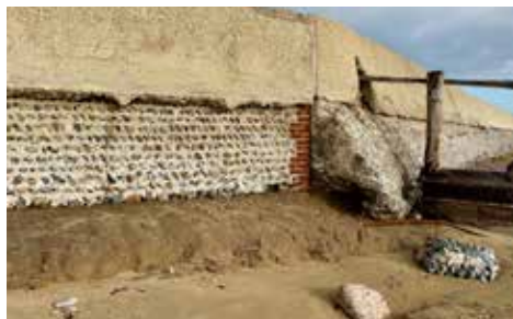
Beach lowering exposes the clay that the original sea defence was built on.
