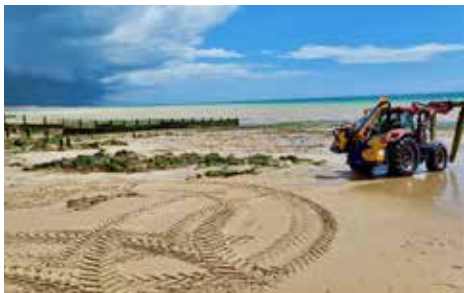
Carrying away a piece of a wooden breakwater. Tracks show where the vehicle has avoided exposed geological features.
