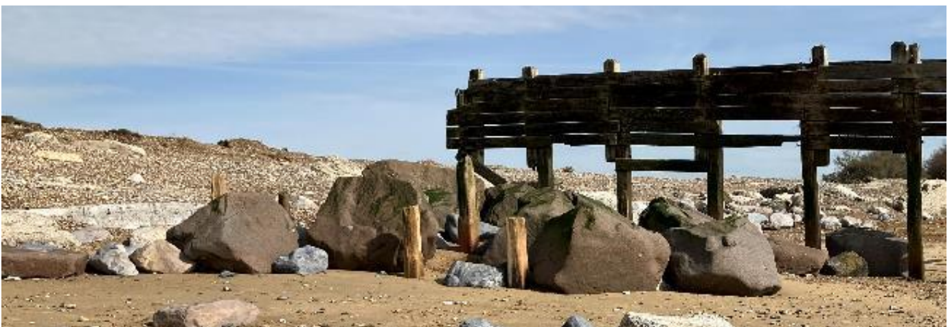
Image two: Large rocks at the head of the groynes east of the car park
