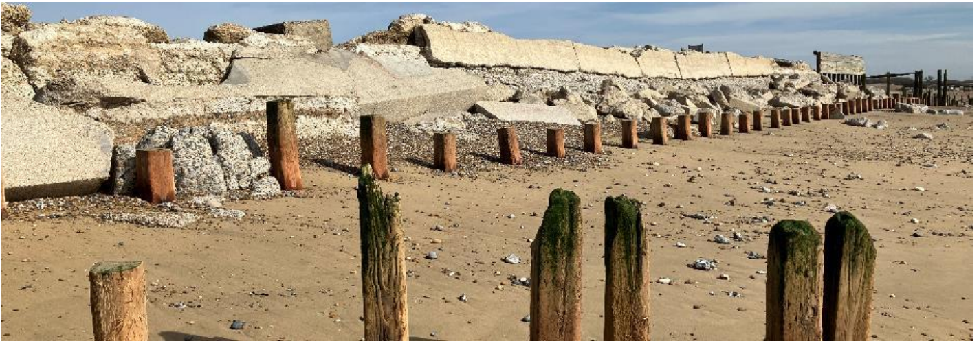
Image one: Wall around western car park
