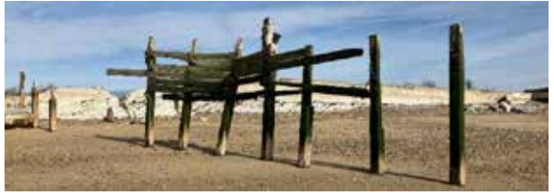
Groyne structure in poor condition and no longer serving a flood risk function
