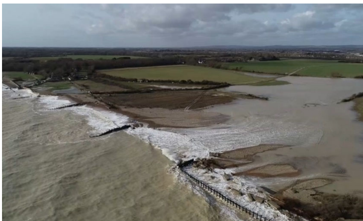
Figure 2 – Breach at Climping frontage in 2020.
