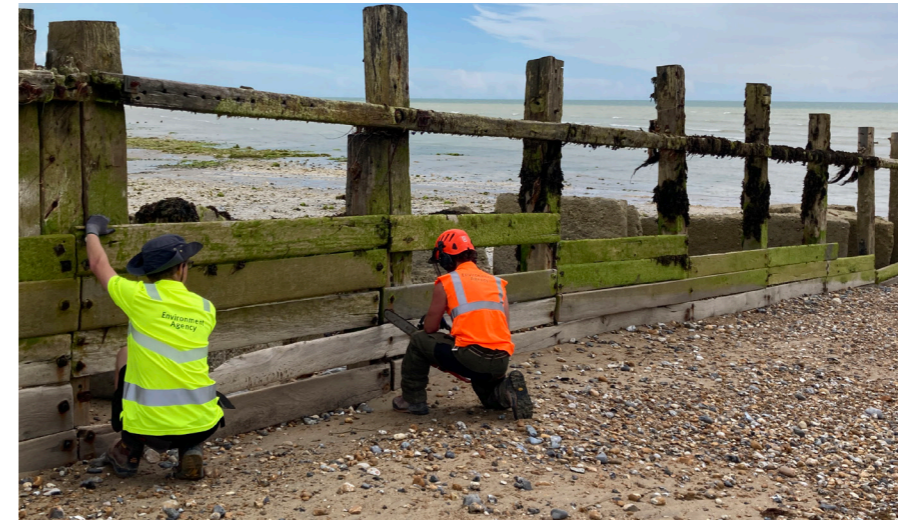
Environment Agency officers conducting groyne maintenance at Climping.
